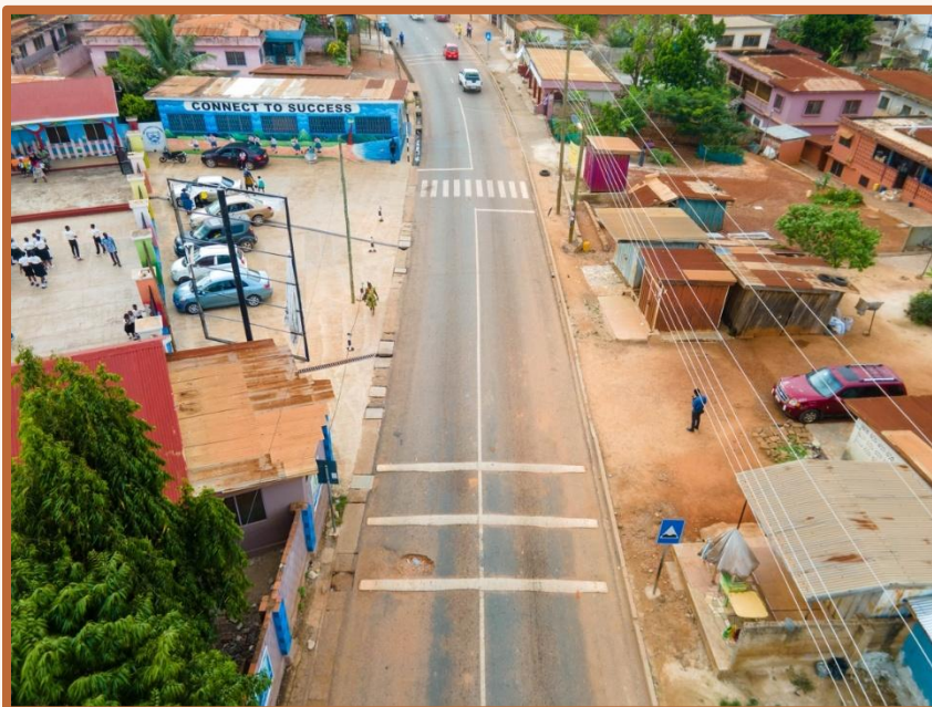
An aerial view showing rumble strips and crossing at the St. Georgie's Basic School
