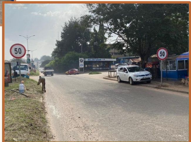
Speed Limit Signs on the Kumasi – Accra Road (Susuanso)
