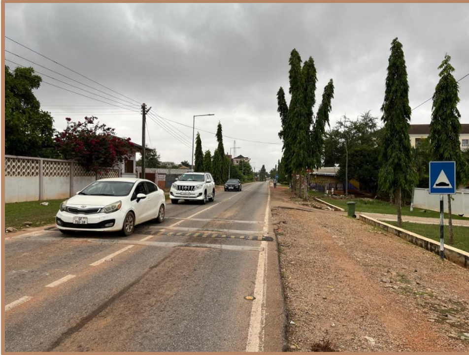
Installed Rumble Strips Along Lesley Opoku-Drive (State Experimental School)
