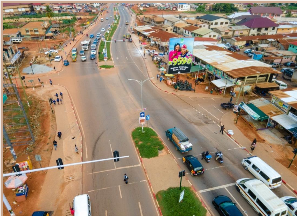
An aerial view showing one of six completed signalized intersections with pedestrian phases along Lake Road
